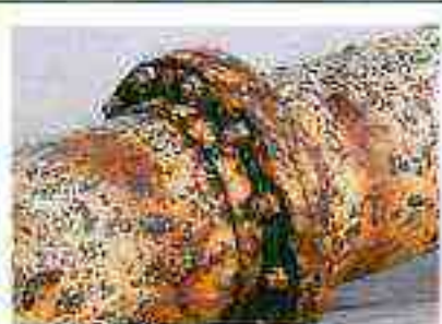
ACOG Grant Services routinely assists communities with grants related to infrastructure repair and improvement.
